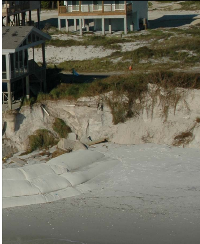
Figure 7. Aerial photograph showing increased dune scalloping around southern terminus of geotubes caused when the geotube return was flanked (289 White Sands Drive visible on the left. Florida Department of Environmental Protection (September 17, 2004)
