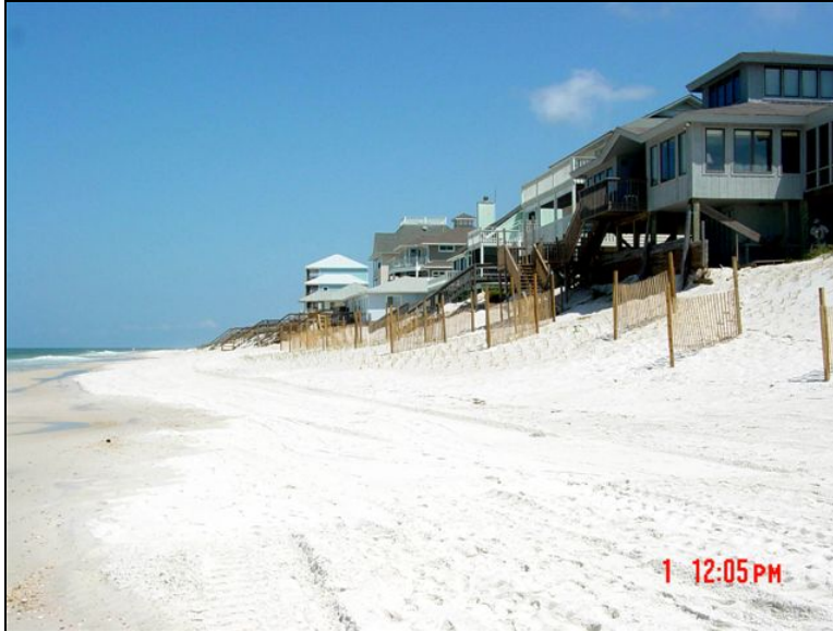
Figure 3. ProTecTube site showing dune rebuilding and re-vegetation upon completion of installation and prior to storm events. 289 White Sands Drive is first house on right. Jay Sample, ACT Inc.
